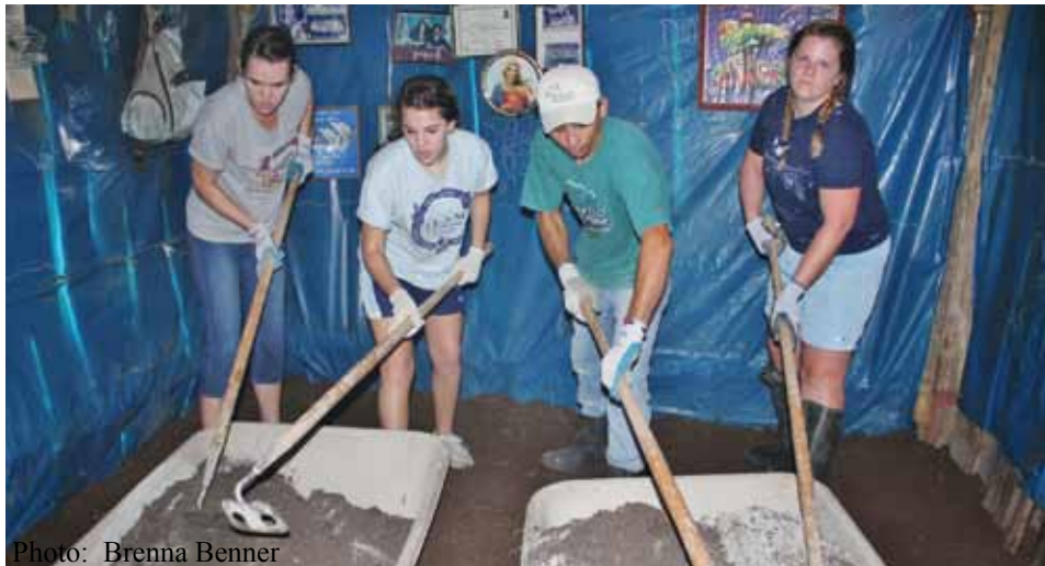
Wilson (middle) working with a visiting team, cementing the floor of a home.
